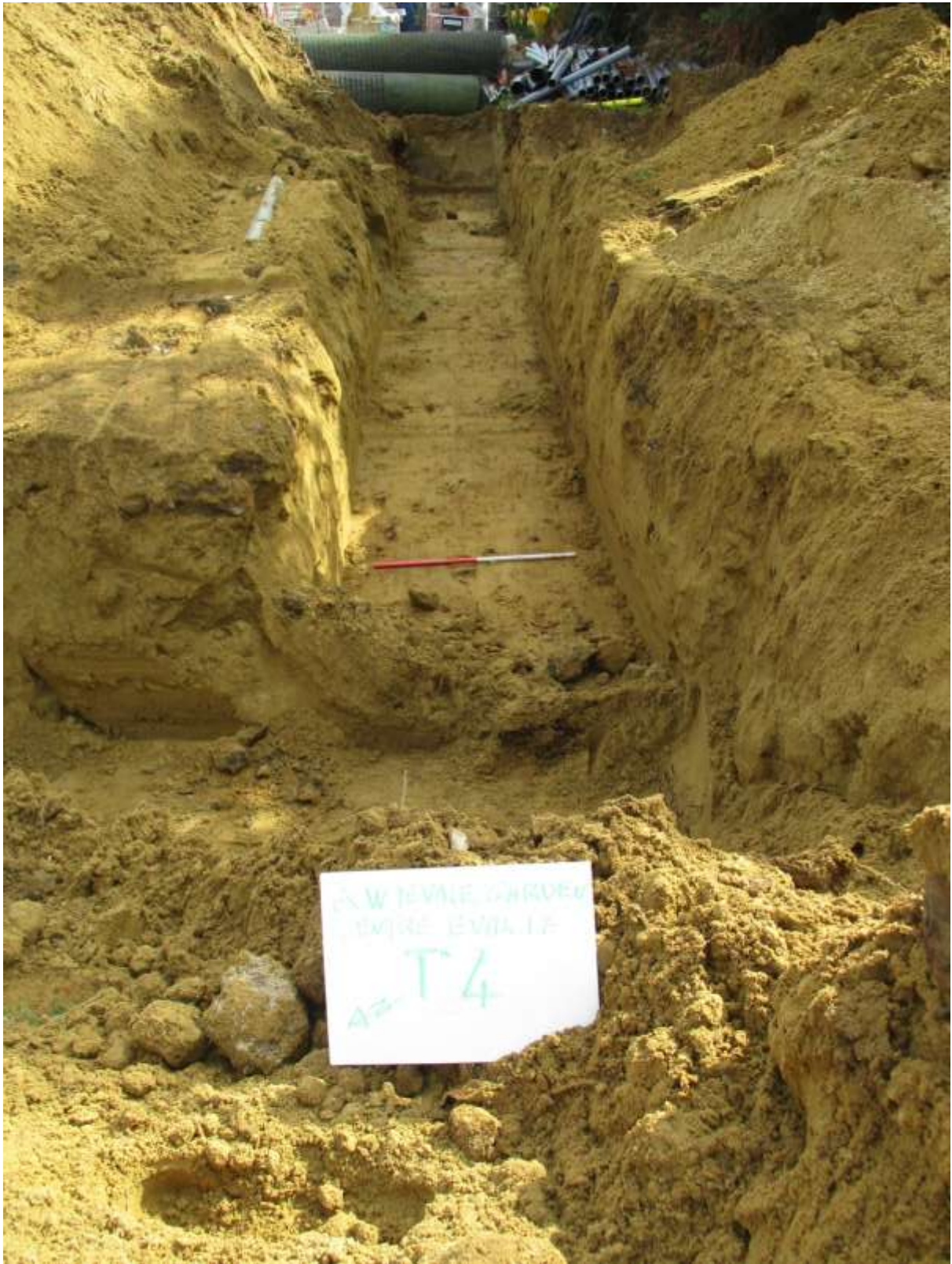
Plate 5. Trench 4 (looking SE)
